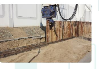
We do all shoring works with sheet piles which are made in many types and sizes. Gulf Foundation specializes in supplying and installing custom hot and cold rolled steel sheet piles.
