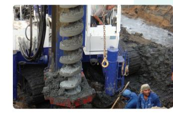
displaced soil as in driven piles and thus, it mostly relies on end-bearing capacity of the earth layer at the drilled depth. Bored piles can provide large pile dimensions and thus high load bearing capacities.
